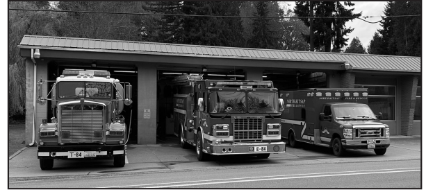
Among the concerns that drive NKF&R's plans to replace the Suquamish fire station are the facility's advanced age and the property's limited size.
